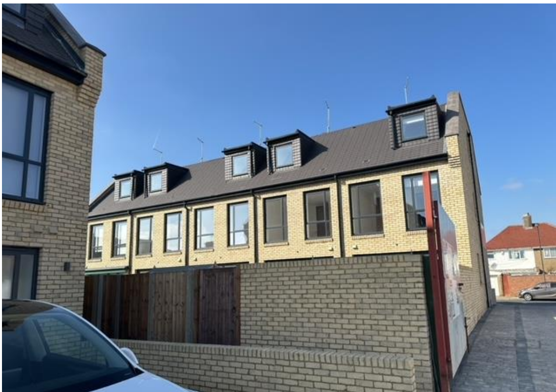
Rear of Block A – built rear dormers
